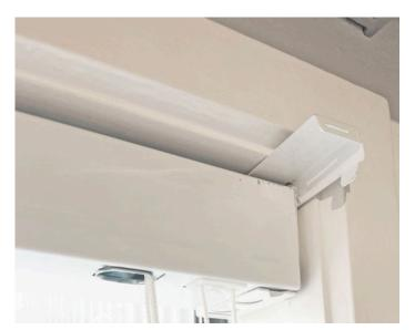
Push the bottom of the bracket upwards and then pull the front out. Repeat with the opposite side.
